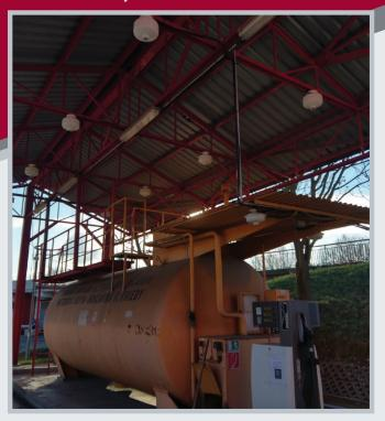
electrical current which activates the unit allowing the fire suppressing powder to be discharged. Each unit has a maintenance free, life expectancy of up to 12 years.None of the components and materials used in the manufacture of the Sapfir system are harmful to the environment.
